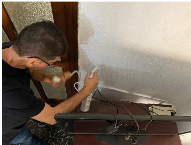
Figure 16 - Domestic interventions. Installing power plugs to reduce consumption
